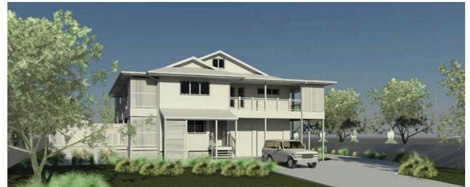
The gambrel roof design has been used to improve the energy efficiency of the home by shading the structure, reducing the cyclone bracing loads and maintaining the country Queensland style aesthetics. The Dutch gables gablet allows for permanent roof venting.
